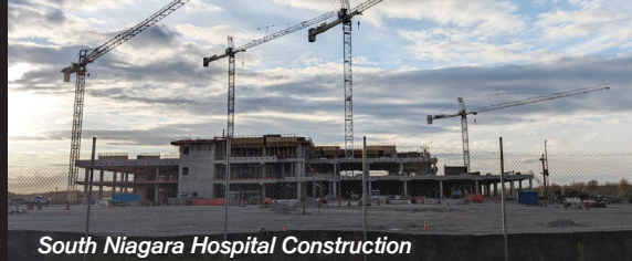
South Niagara Hospital Construction
